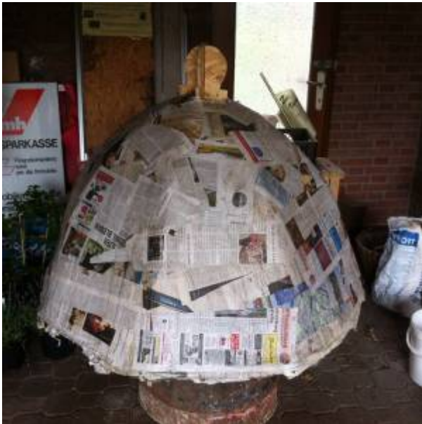
Turmhelm in Bau
